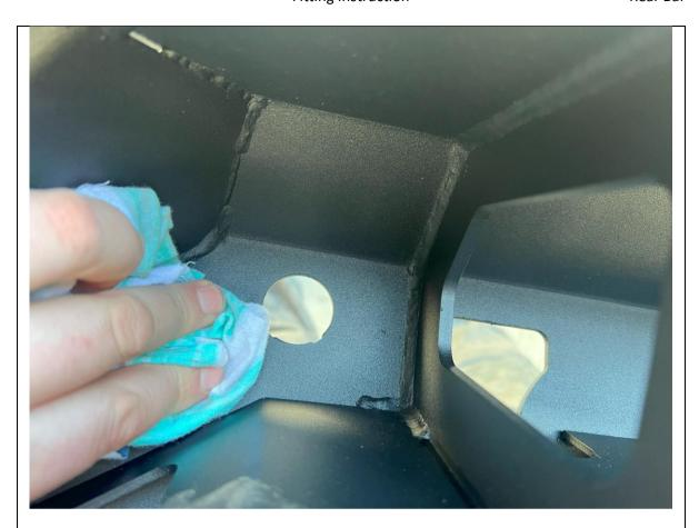
14. Clean areas adjacent to parking sensor locations on inside of bar with isopropyl alcohol.
